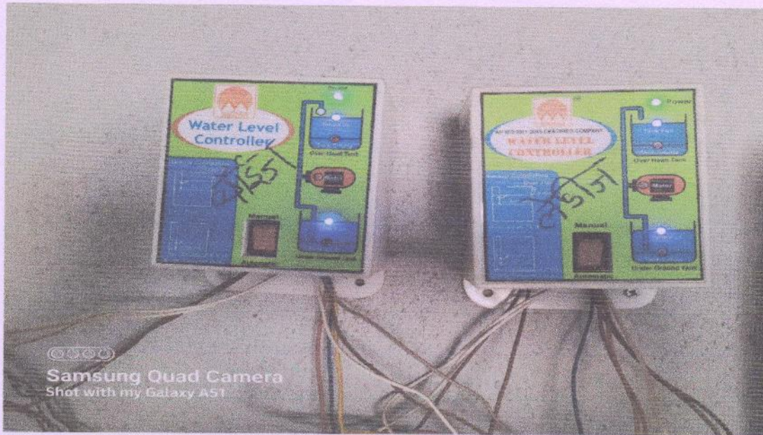
Sensor base automatic on / off for water tanks
