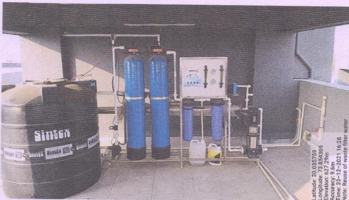
Ro Water Purifier & its residual waste water collected in tank & also utilized for gardening purpose
