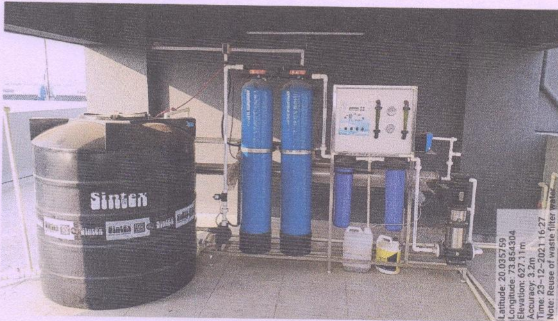
Ro Water Purifier & its residual waste water collected in tank & also utilized for gardening purpose
