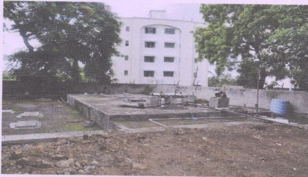
Water Tanks in college campus
